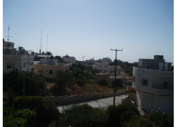
(Picture 6.3) Two to three story buildings (source: the researcher)
